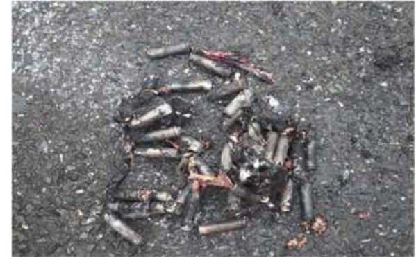
Burn damage status of lithium-ion batteries
